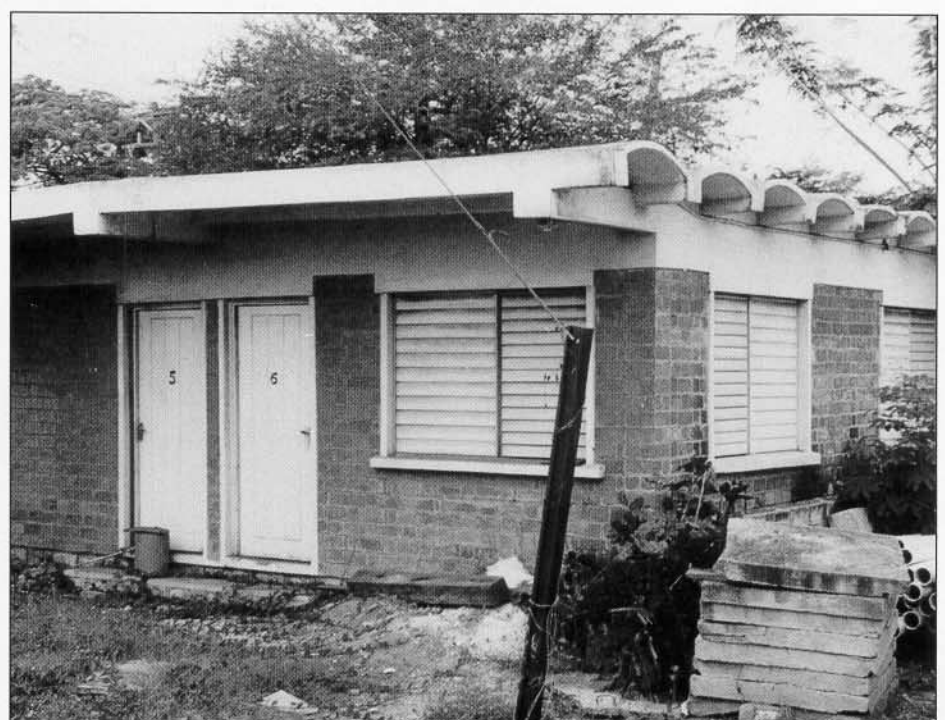
Fig. 4: The BRI red mud demonstration building (1998)
