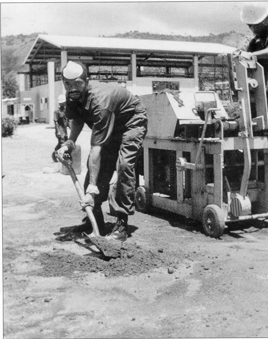
Fig. 3: Wet mixing of raw materials just before pressing
