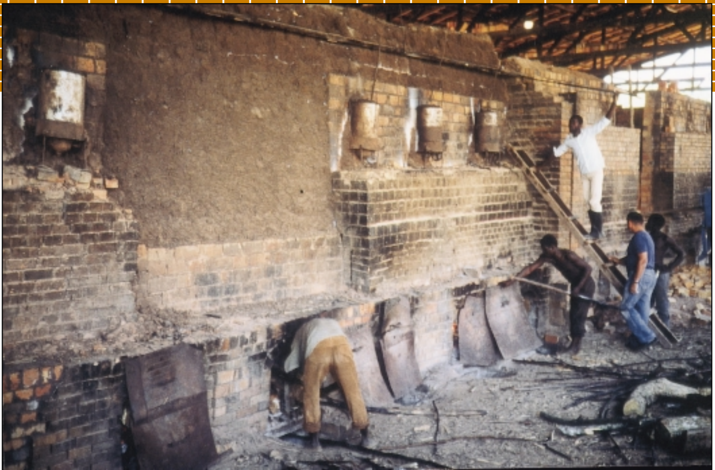
Fig. 3: Combined firing system: Firewood is fed on the bottom. Coffee husks are fed from above. Fire holes are covered with pieces of sheet-metal
