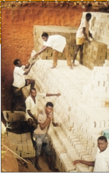
Fig. 4: Clamp dug into sloping ground
