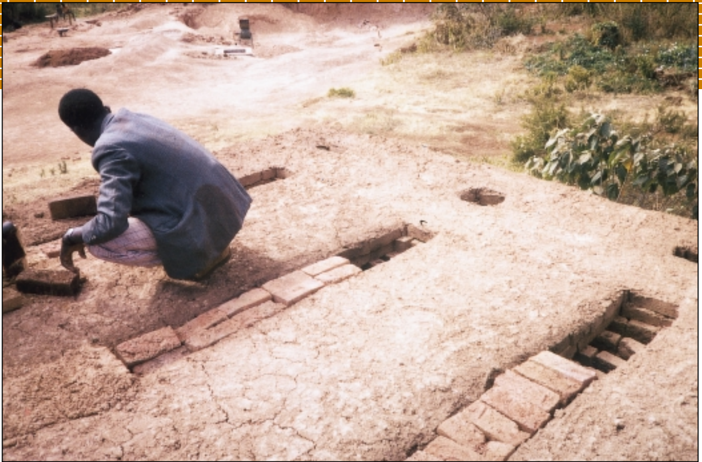
Fig. 1: Sealing of the clamp's top against heat loss; leaving smoke outlets
